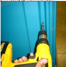
Drive fourth lag screw into rear panel dimple left of the 3<sup>rd</sup> lag 19-3/4" [50.17cm] and 16-1/2" [41.91cm] up from the floor.
