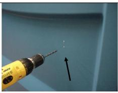
Place 7" [17.78 cm] tube P/N 15589 in short end of one handrail P/N 18038 with at least 3.5" [8.89 cm] left sticking out. Drill #10 hole through handrail into tube. Install #68 STNLS rivet PN #11270.
