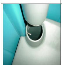
Drive third lag screw through rear panel into dimple in groove to tank and vent pipe at 17-1/2" [44.45cm] up from the floor.
