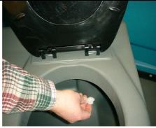
Phillips driver bit and drill can be use to tighten. Be careful not to over tighten nut.
