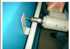
Install 3/16" Fender washer PN 11361 and 3/16" backup washer PN 11315 on outside of panel and set rivet.
