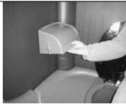
**Finish paperguard installation.**Drill the four dimples shown for the paperguard using a #10 (0.194") drill bit. (use drill stop to prevent drilling through outside wall.)
