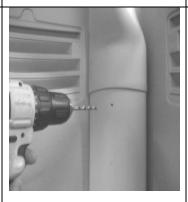
Using a silver colored expanding rivet PN 17436, attach the coat hook to the vent pipe.
