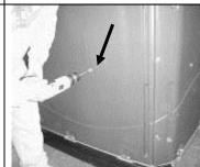
Install screw to hold bottom spring arm between base & panel.
